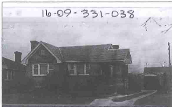
1615 E. Harvard Ave. Built 1925 Striated brick, stucco/plaster Bungalow
