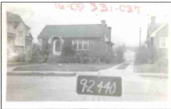
1611 E. Harvard Ave. Built 1925 by Herrick Bros. Striated brick with half timbering, Bartile roof English Tudor Bungalow
