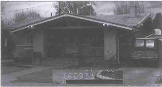
1553 E. Harvard Ave. Built 1915 by H.J. McKean Stucco/plaster, shingle siding Arts & Crafts Bungalow
