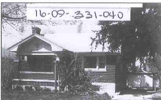
1627 E. Harvard Ave. Built 1925 by Herrick Bros. Regular brick with half timbering Bungalow Queen Anne
