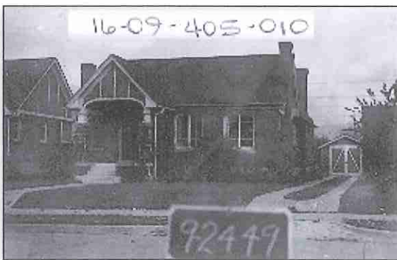
1659 E. Harvard Ave. Built 1926 by Herrick Bros. Regular brick with half timbering English Tudor Period Cottage
