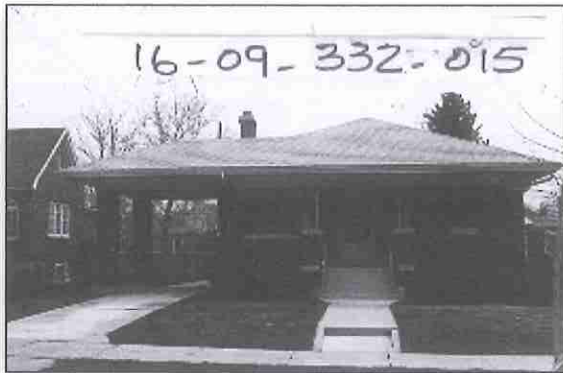
1590 E. Harvard Ave. Built 1920 by Builders Loan & Trust Stucco/plaster, stone veneer Prairie School Bungalow
