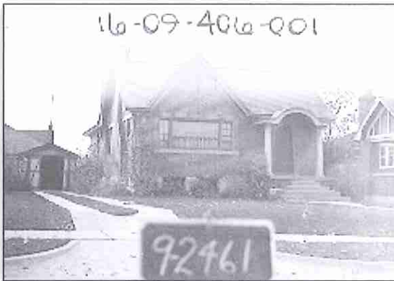
1656 E. Harvard Ave. Built 1926 by Herrick Bros. Striated brick with half timbering English Tudor Neoclassical
